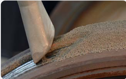
Suction nozzle butt weld
