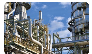
Anlagenbau | Plant construction
