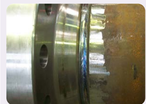
Tube-flange connection welded with manual SAW equipment
